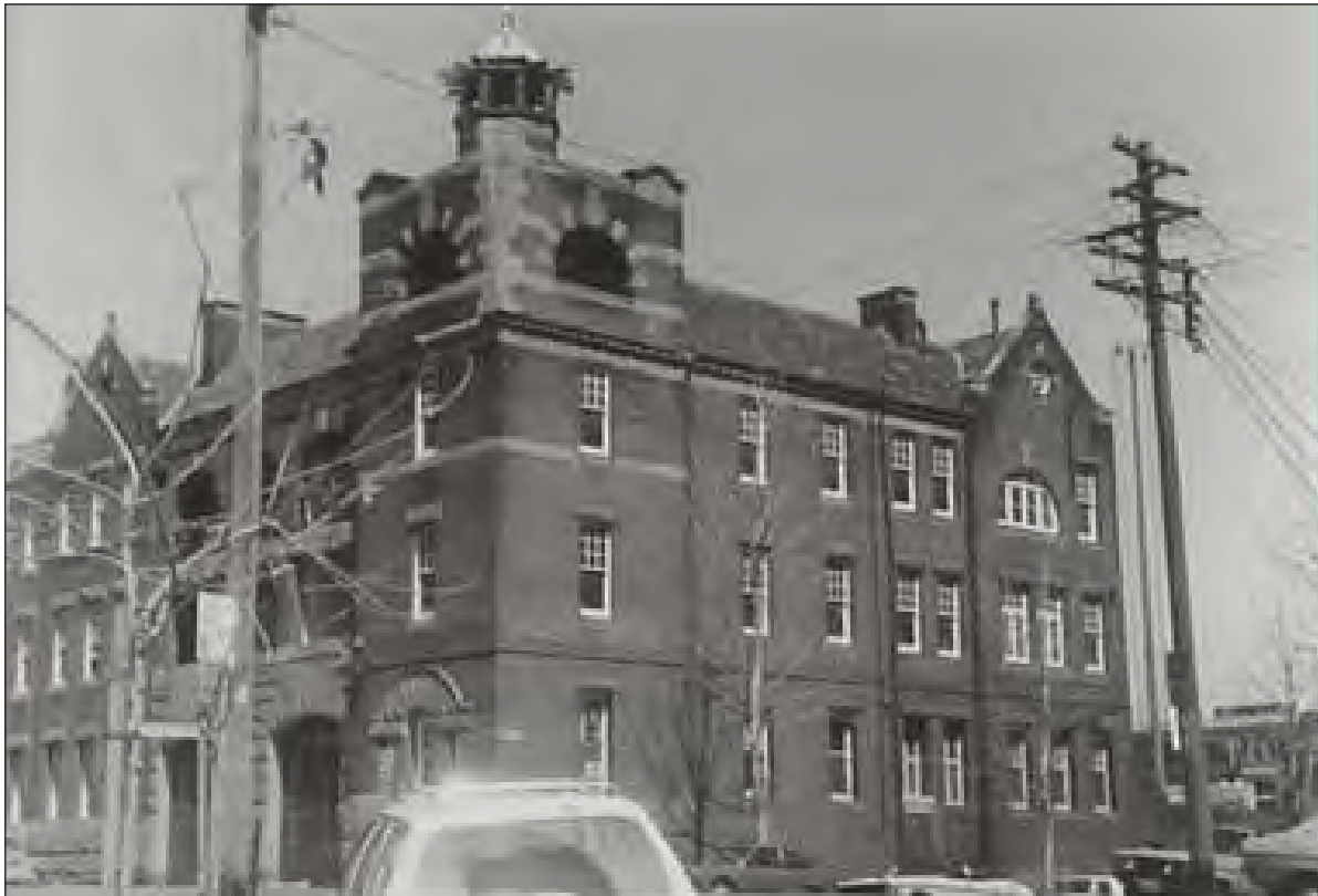
Pymont Fire Station, 1979. 41
