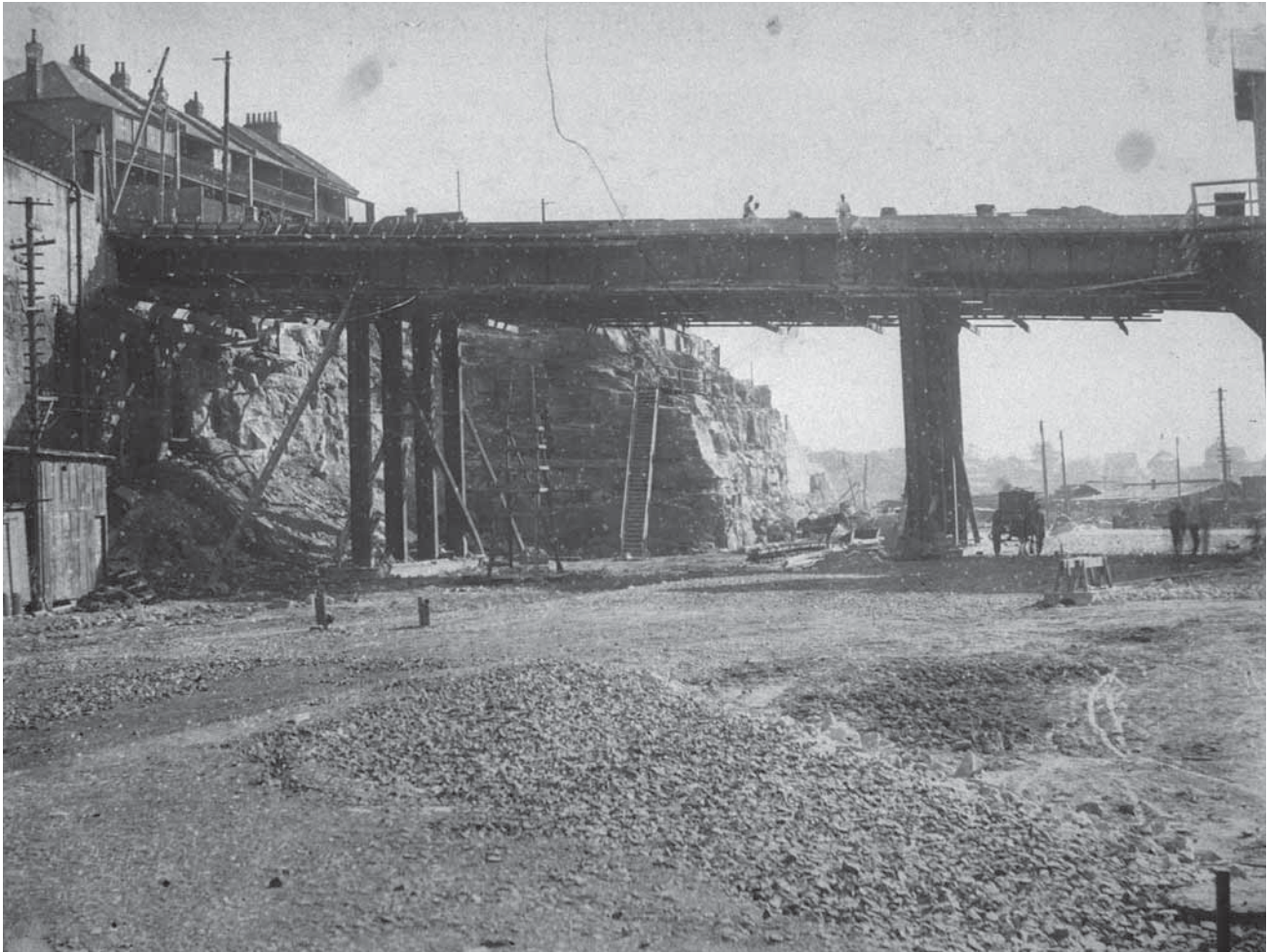
Figure 5.5.5: Anon, 1917, Construction of overhead bridge to Jones Bay wharf (ML Government Printing Office GPO 1_24482/digital order no. d1_24482)
