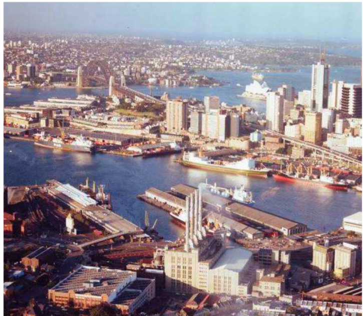
Pyrmont 'B' Power Station. Aerial view of power station and associated buildings
