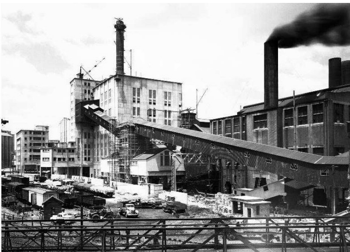
Pyrmont 'A' Power Station. Poor chimney stack emission from inefficient chain-grate boilers
