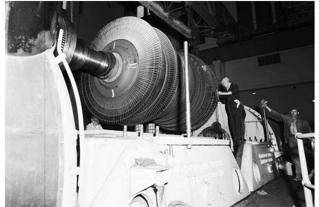
Pyrmont 'B' Power Station. Turbine Rotor Overhaul
